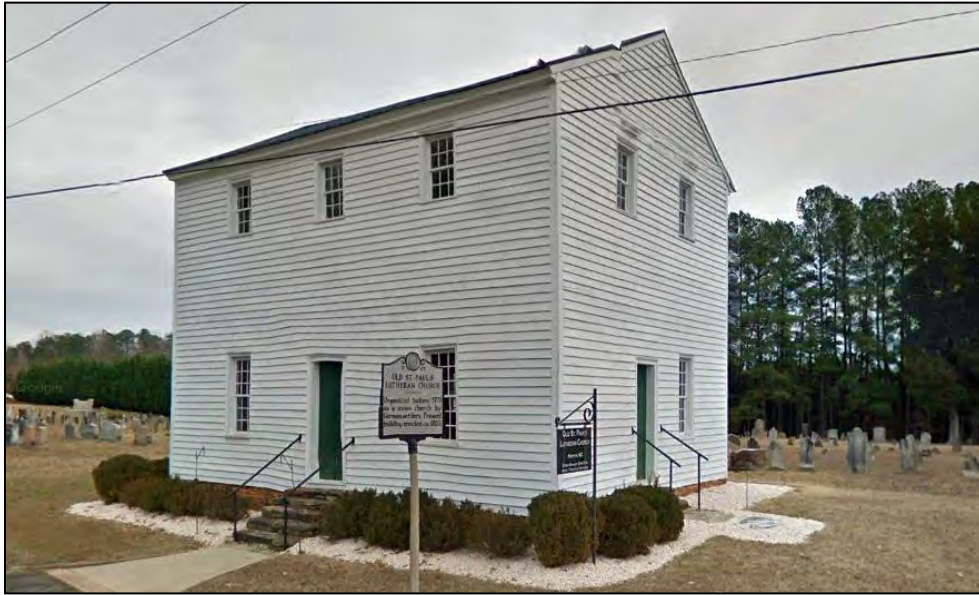
Photo 42: Old St. Paul's Evangelical Lutheran Church, Original Circa-1818 Building, Southwest Oblique.
