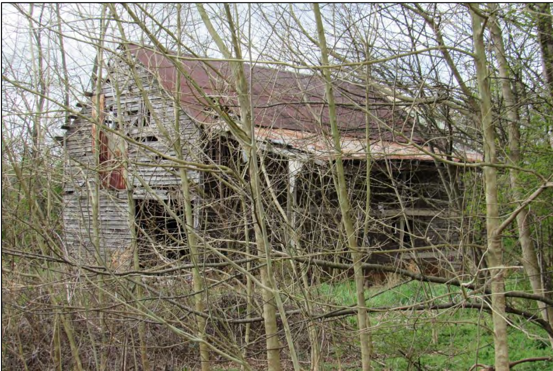
Photo 7: Second Barn on the W.R. Lutz Farmsite, Northwest Elevation.
