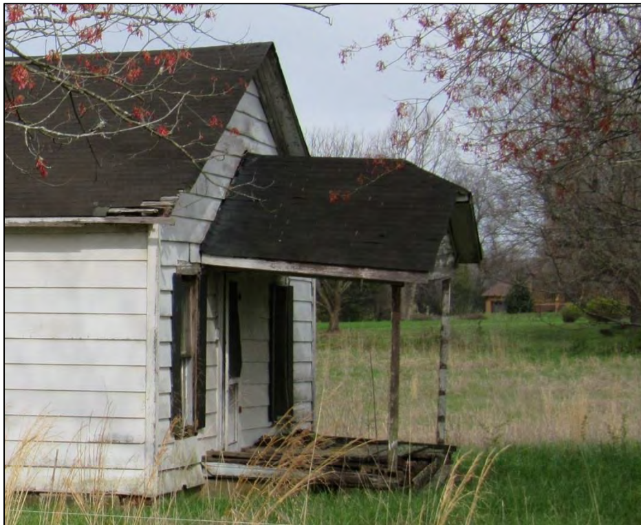
Photo 3: Tenant House Porch Detail, Looking North.
