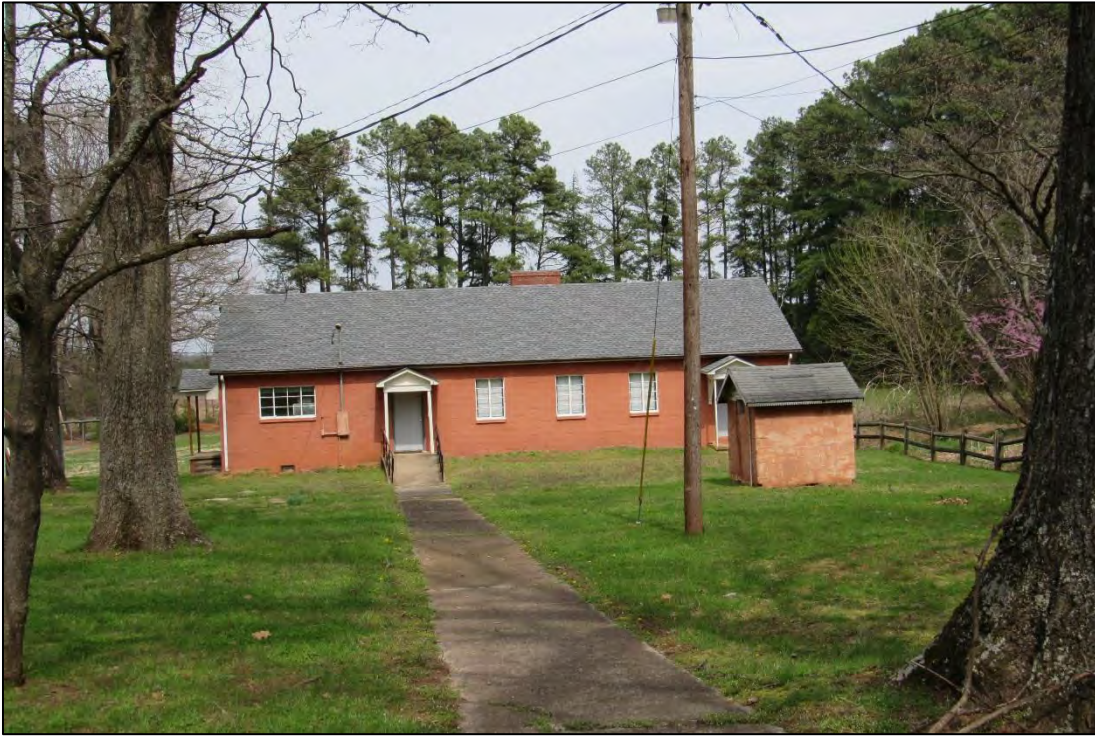
Photo 36: Trinity Hmong Lutheran Church, Education Building, Primary (Southwest) Elevation.
