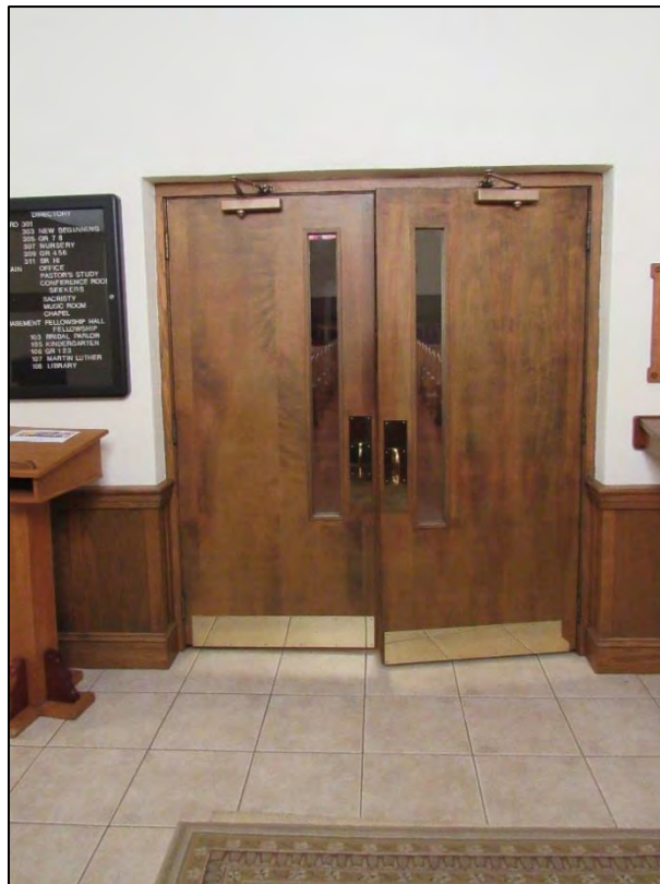
Photo 26: Example of Replacement Flooring in St. Paul's Lutheran Church.
