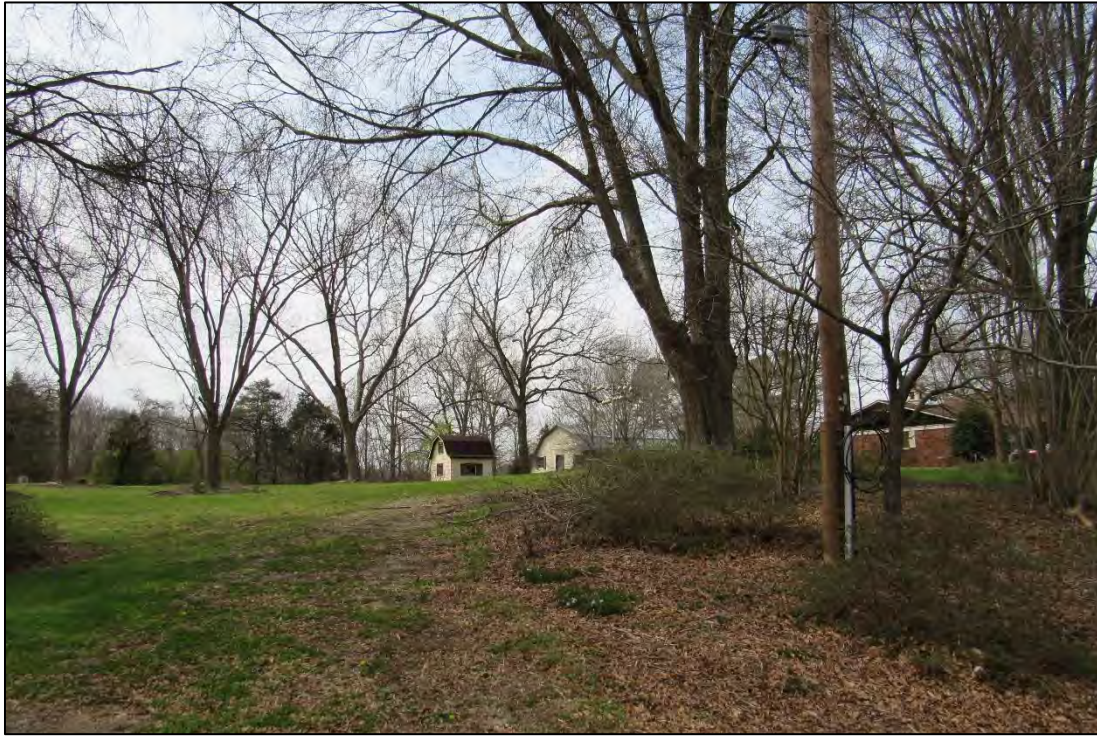
Photo 17: Historic Dairy Outbuildings to West of Main House, Facing North.
