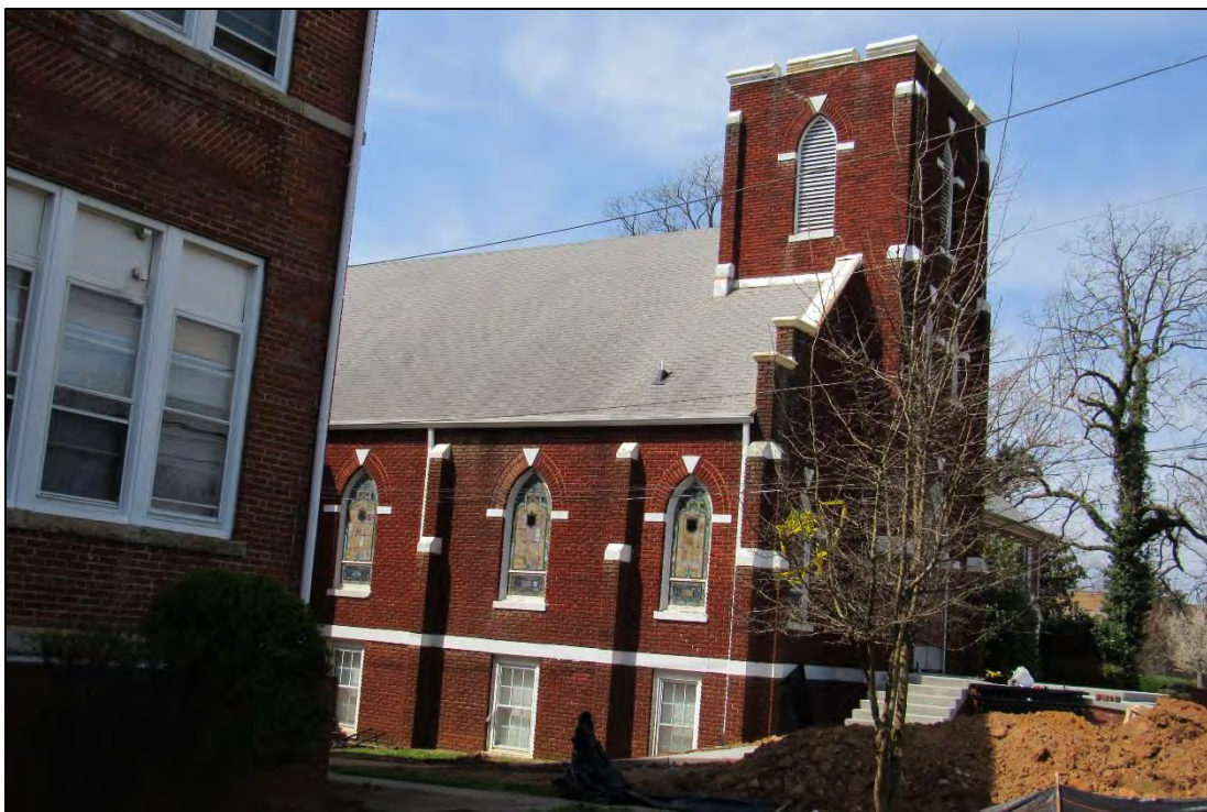
Photo 30: Christ Lutheran Church, Detail of South Elevation.
