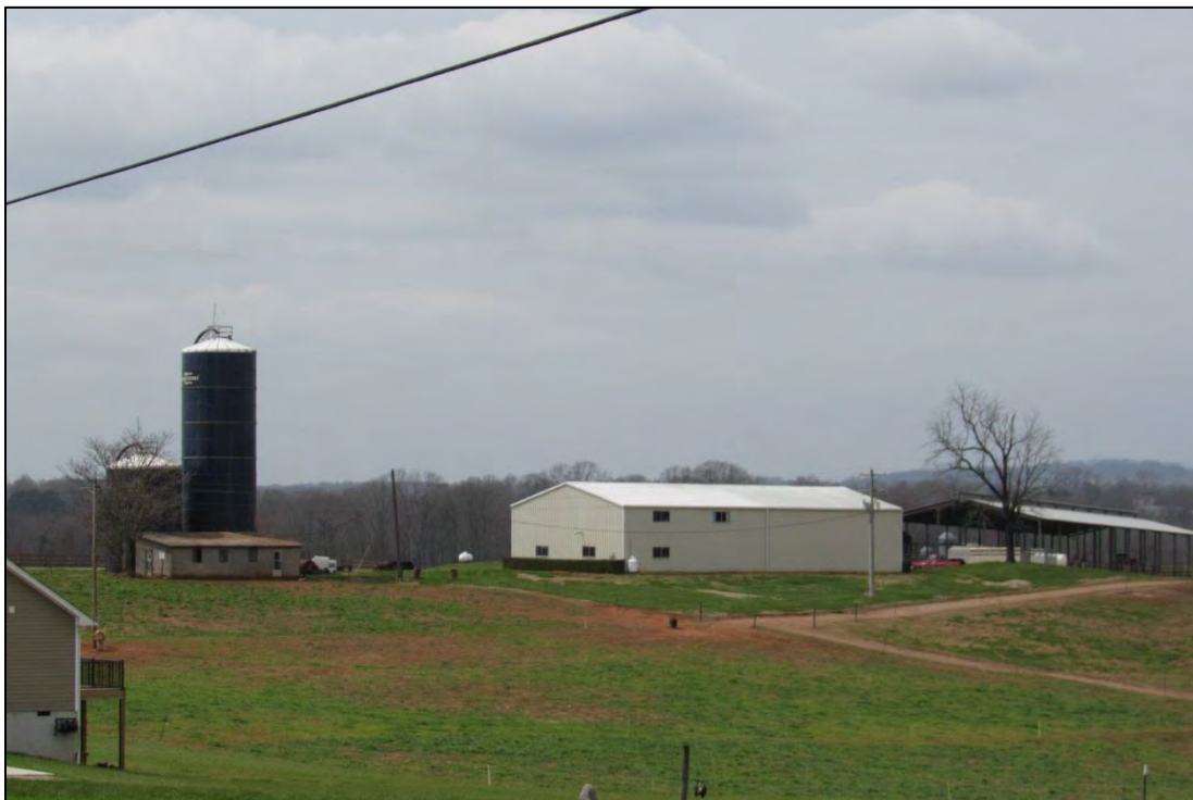
Photo 12: Detail of Silos, Barn, Milking Parlor, and Equipment Shed, Looking West.
