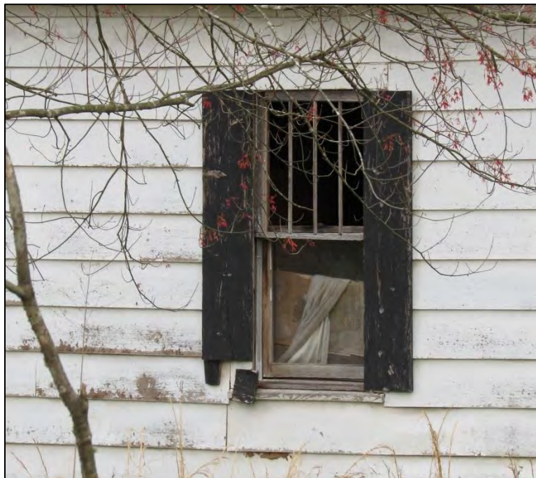
Photo 5: Example of Original Four-Over-One Wood Window, Southeast Elevation.
