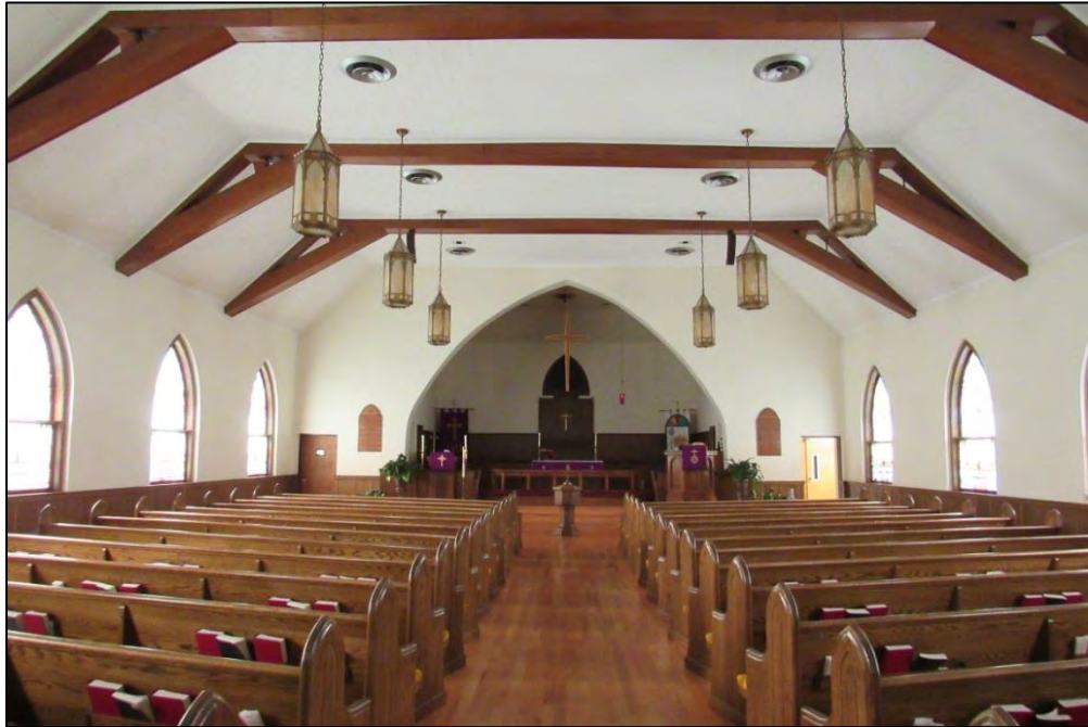
Photo 25: Interior of Nave in St. Paul's Lutheran Church, Looking West Towards Chancel.
