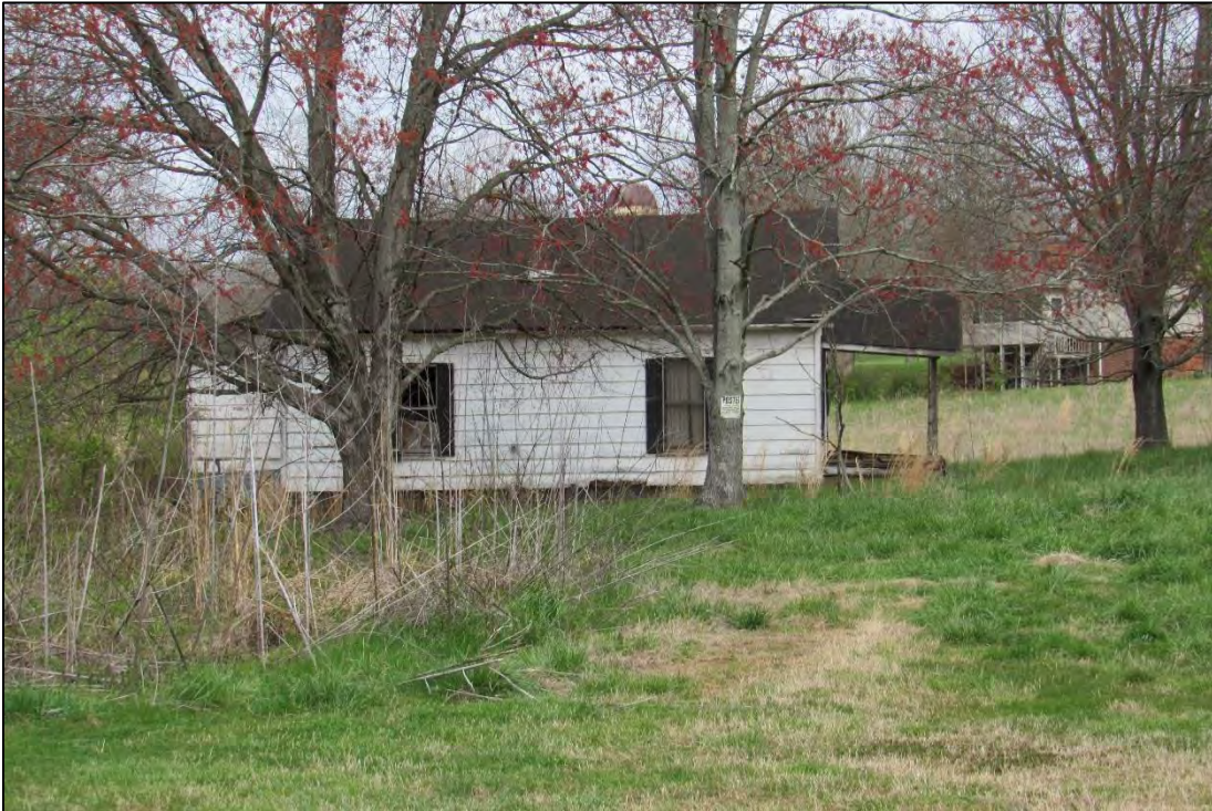
Photo 2: W.B. Lutz Tenant House, Southeast Elevation.
