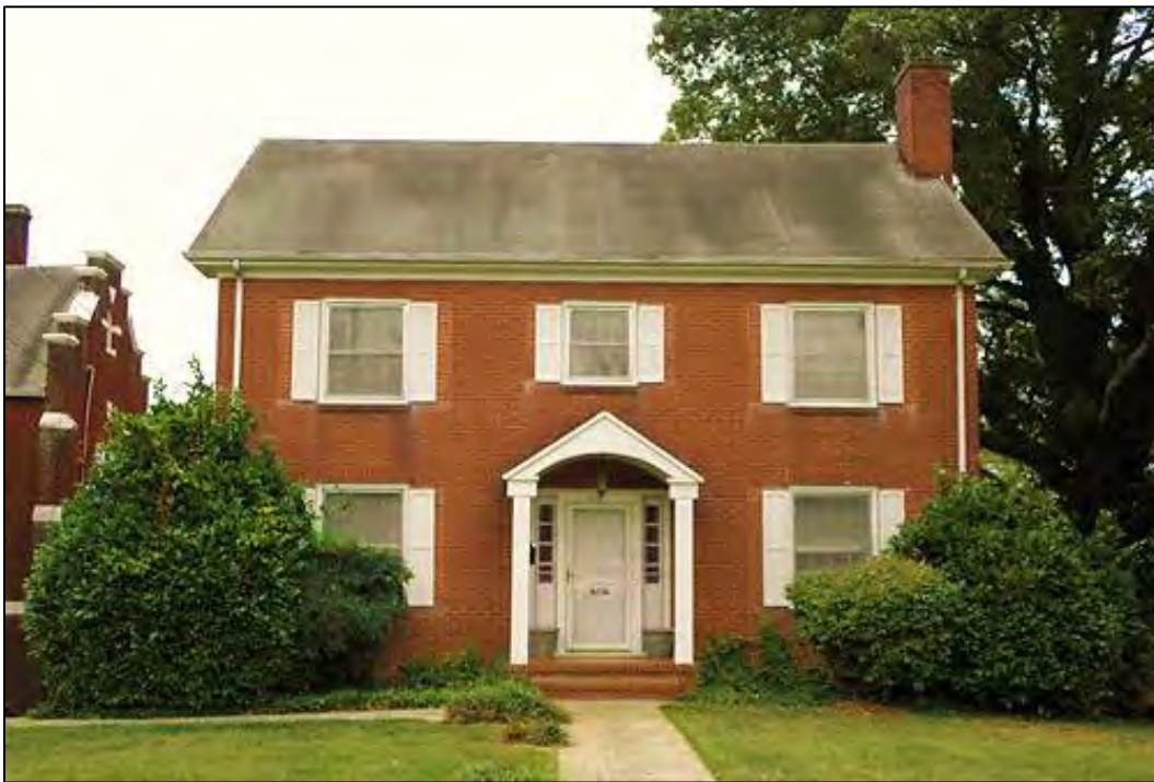
Photo 32: Parsonage at Christ Lutheran Church, Primary (West) Elevation.
