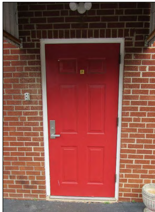
Photo 24: Replacement Door on St. Paul's Church Addition.
