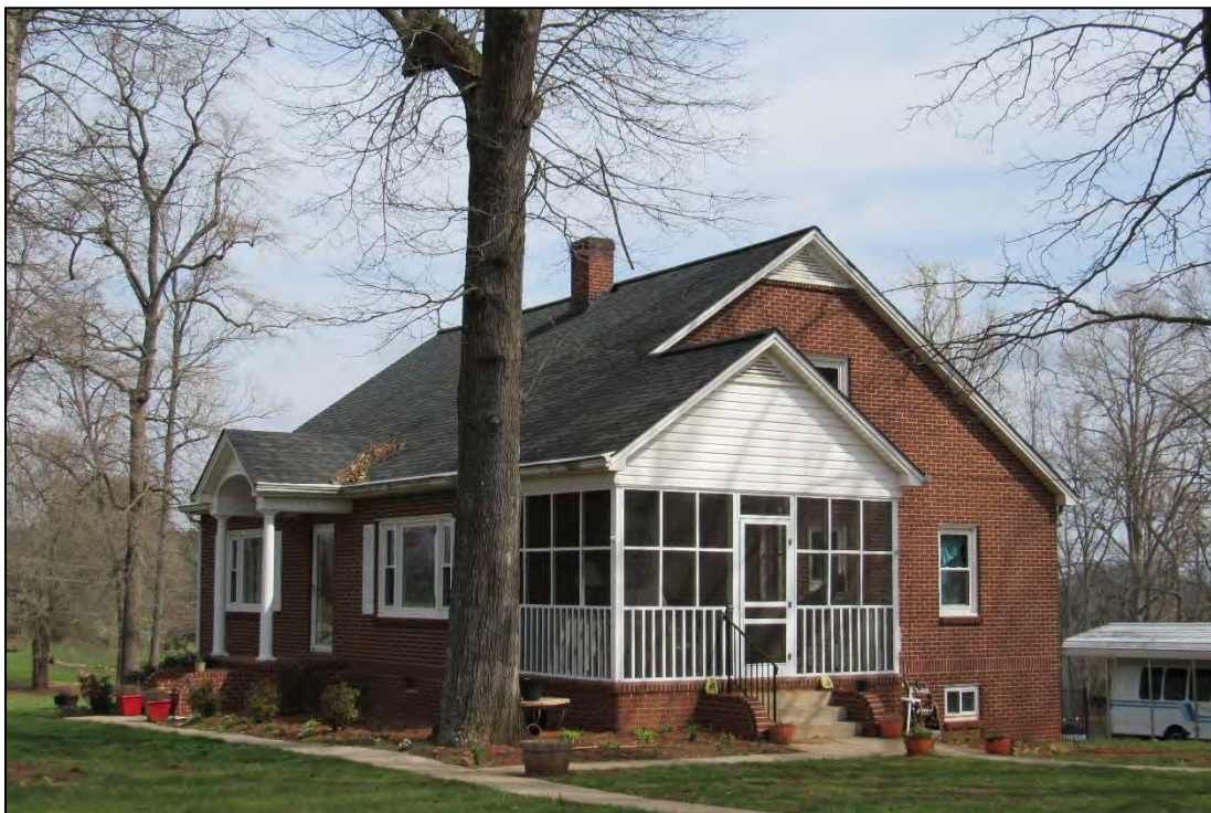
Photo 41: Grace Lutheran Church Parsonage, Southwest Oblique.
