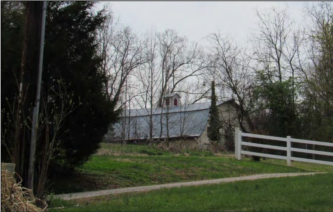
Photo 19: Additional View of Dairy Barn, Facing Southwest.
