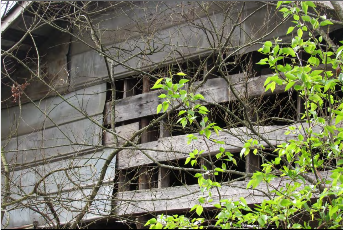
Photo 8: Detail of Framing on Second Barn, Looking Southwest.
