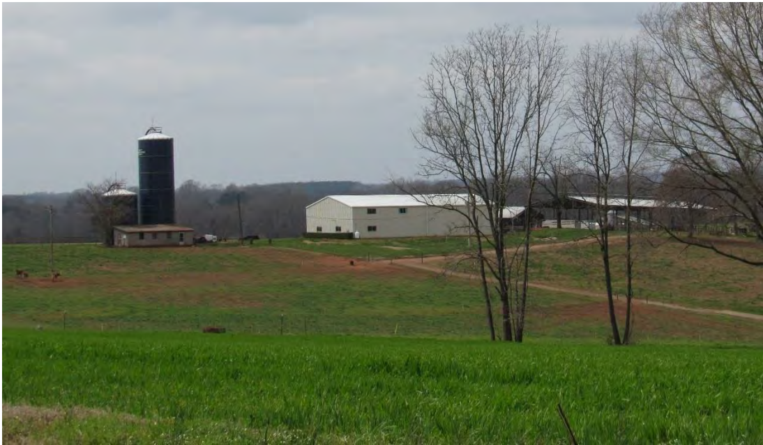
Photo 11: Overview of Modern Dairy Buildings, Looking North.
