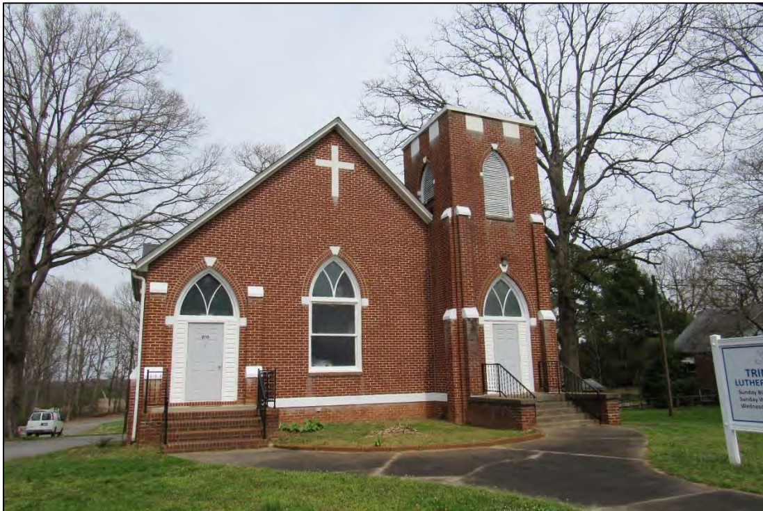
Photo 34: Trinity Hmong Lutheran Church, Primary (Southwest) Elevation.
