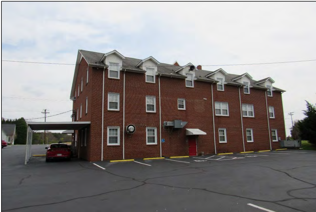
Photo 21: Rear (East) of Addition on St. Paul's Lutheran Church.
