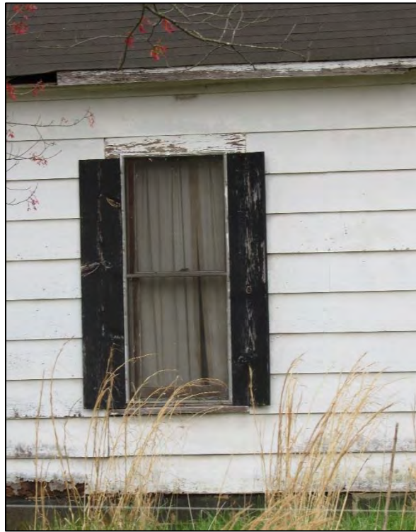
Photo 4: Example of Aluminum-Framed Replacement Window, Southeast Elevation
