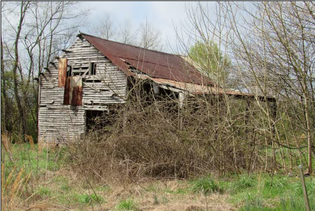
Photo 6: Second Barn on the W.R. Lutz Farmsite, South Oblique.
